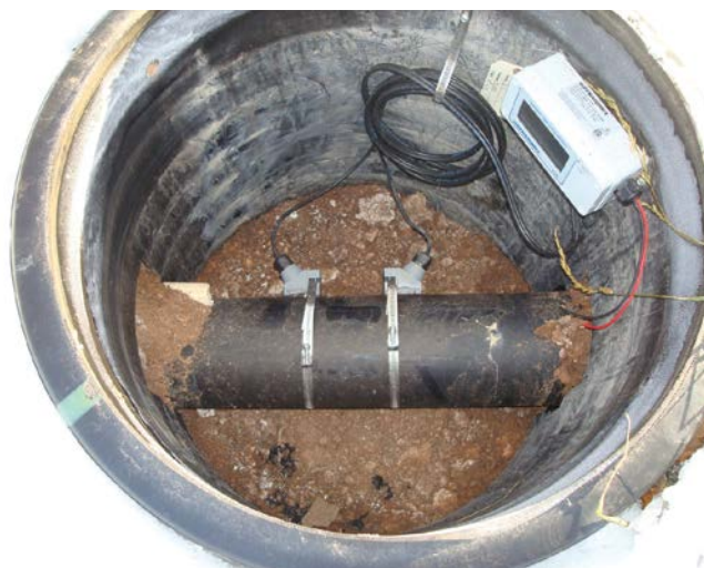
The transit-time flowmeters use strap-on transducers, which function as ultrasonic transmitters and receivers.
