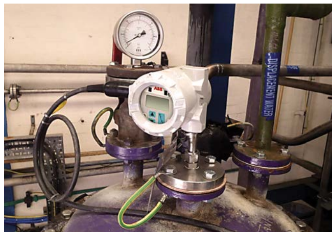
Figure 2. U.K.-based Robinson Brothers is using a magnetostrictive level transmitter from ABB to meet strict safety standards for handling highly reactive carbon disulfide ( \text{CS}_2 ).
