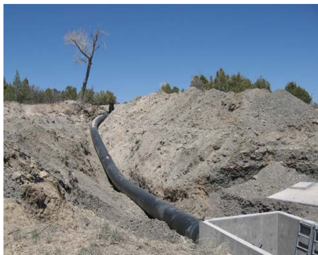
In this pilot project, open ditch irrigation canals were replaced with a closed water distribution system. It reduces evaporation, cuts seepage and eliminates end-of-channel water losses.
