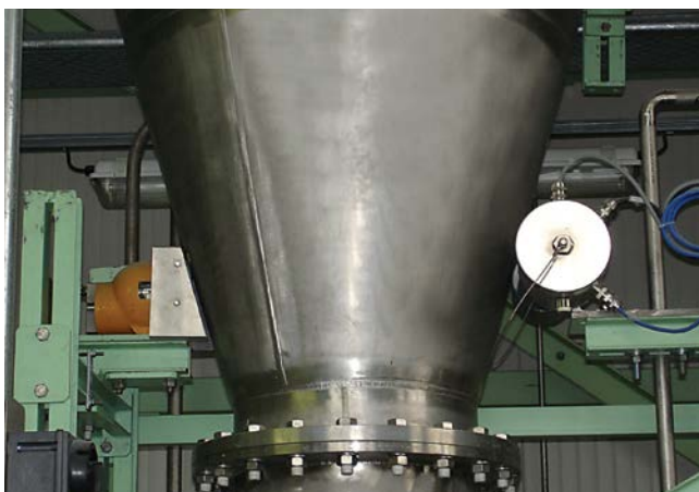
POINT LEVEL SWITCH IN A HOPPER
